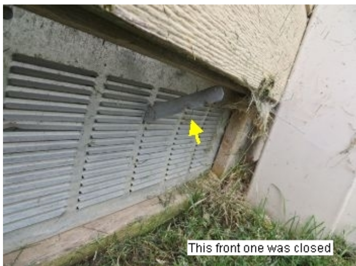
BE sure to have crawlspace vents open during summer
