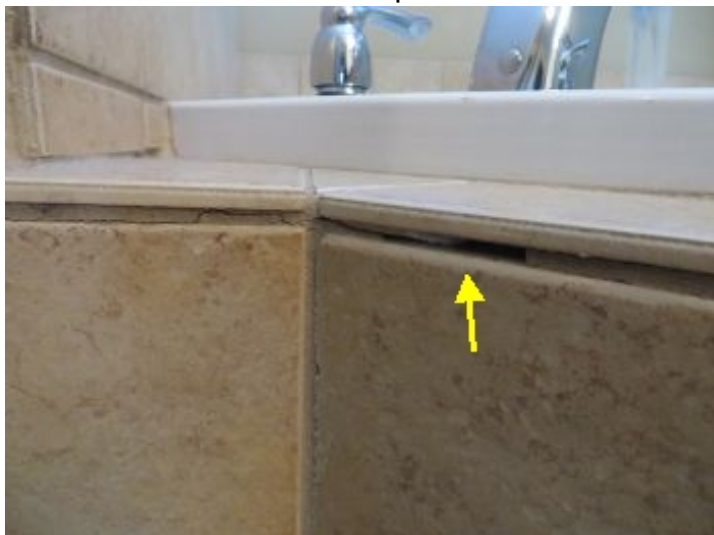
Tub tile has some damaged and missing grout in areas. See photos
