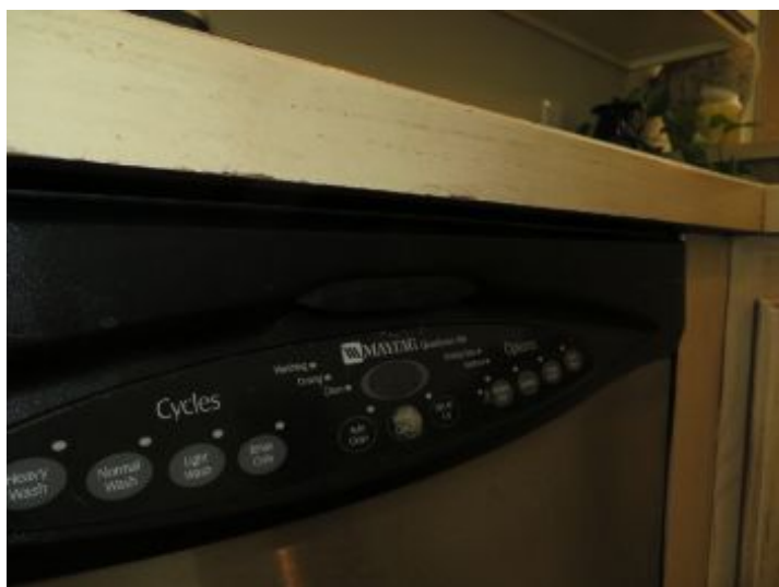
Dishwasher buttons worn and handle can be difficult to open
