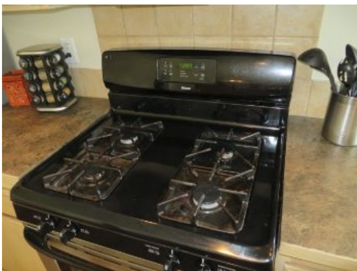
Safety Hazard- Stove Missing anti-tip brackets. This is needed to prevent injury or death. Recommend install prior to moving in.
