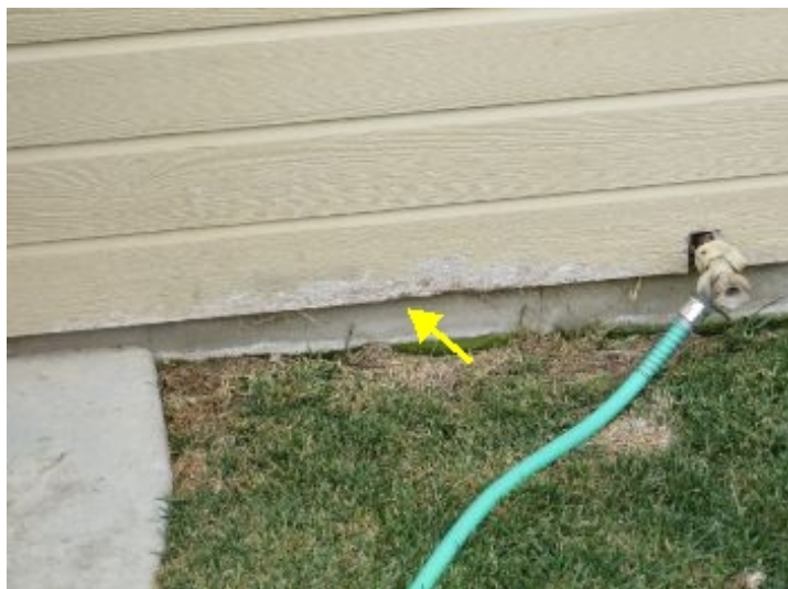
Som lower edge siding is damaged on back of home
