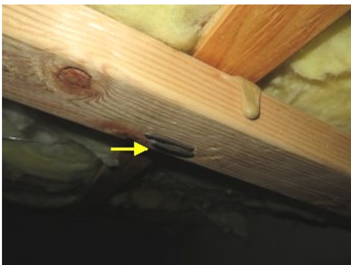
Nail where support used to be
