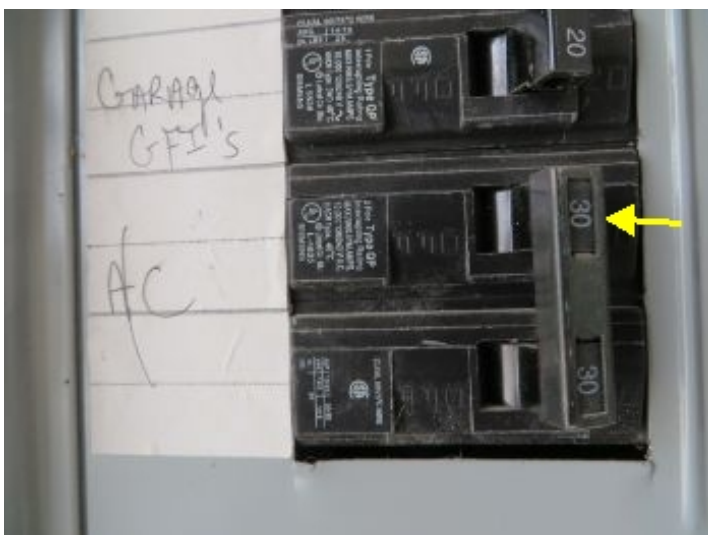
AC breaker in main panel 30amp
