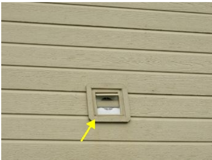
Exhaust fan vents are damaged at the back home. one is missing flaps and other is partly sealed and missing flaps.
