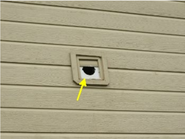
Exhaust fan vents are damaged at the back home. Exhaust fan vents are damaged at the back home. one is missing flaps and other is partly sealed and one is missing flaps and other is partly sealed and missing flaps.
