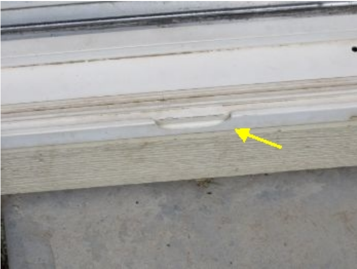
Sliding Door exterior mold of frame has a piece broken off. This is cosmetic only and does not affect the function. See photos.
