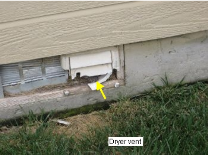
Exhaust fan vents are damaged at the back home. Exhaust fan vents are damaged at the back home. one is missing flaps and other is partly sealed and one is missing flaps and other is partly sealed and missing flaps.
