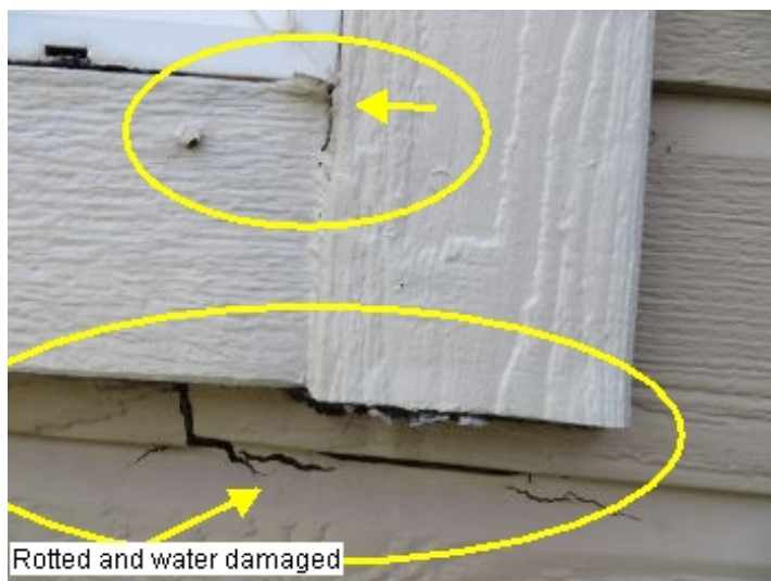
Siding under kitchen window is water damaged (rotted) at the corner. See photos. Can not determine amount of water damage internally. Recommend repair.
