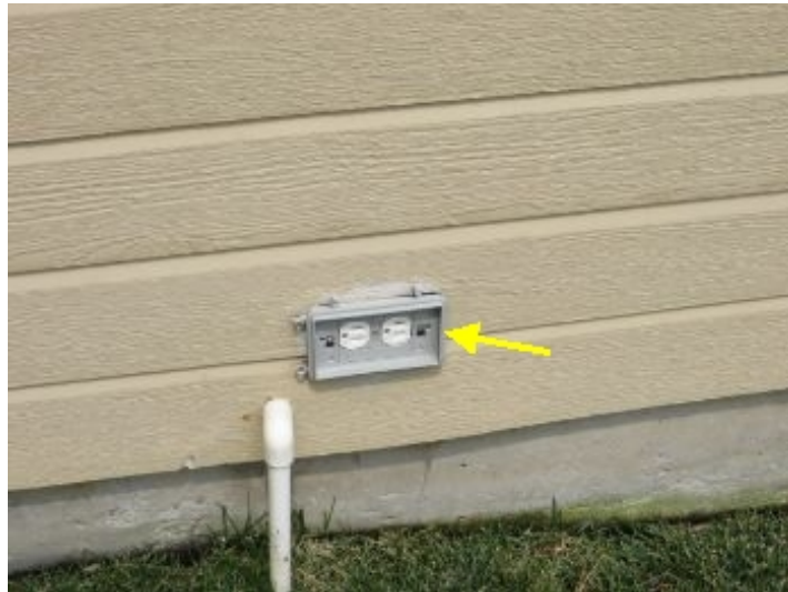
Exterior Outlet cover behind garage damaged.
