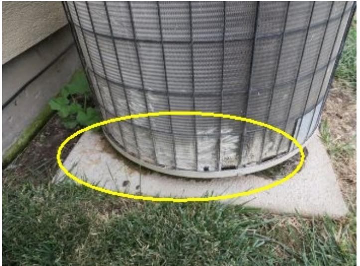
AC Unit on exterior has fin damage. This can reduce the efficiency of the unit, however the unit showed good register temperatures under Thermal Infrared imaging (54-58 degrees) at time of inspection which indicates no loss of efficiency. If unit does not run efficiently during summer, this may be the reason. Recommend consulting with HVAC contractor for repair estimates if needed. Use caution when mowing and weed eating.
