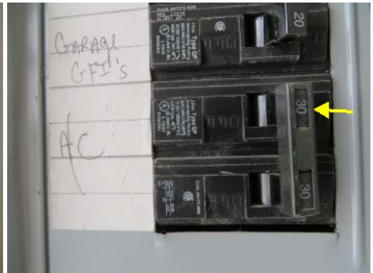
AC breaker in main panel 30amp
