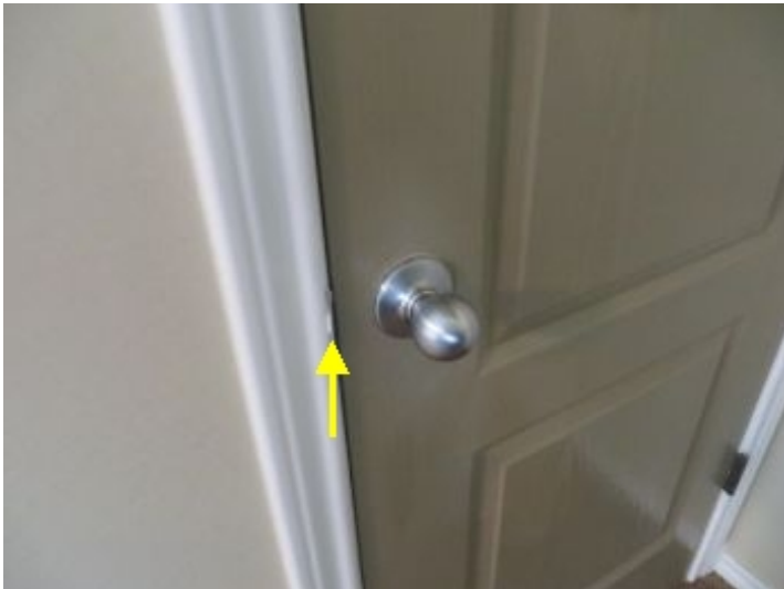
Front entry closet Door striker plate Adjustment needed, Door doesn't latch properly.
