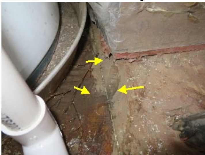
Condensate drip line is likely plugged. There is a large amount of water coming out of the corner of the furnace bottom and none coming out the condensate drip line. This needs repair
