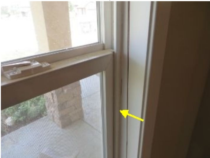
Entry Family Room front right window (from inside home) does not function correctly. Binds and is loose. tracks move and appear to be damaged. Consult with window contractor on repair
