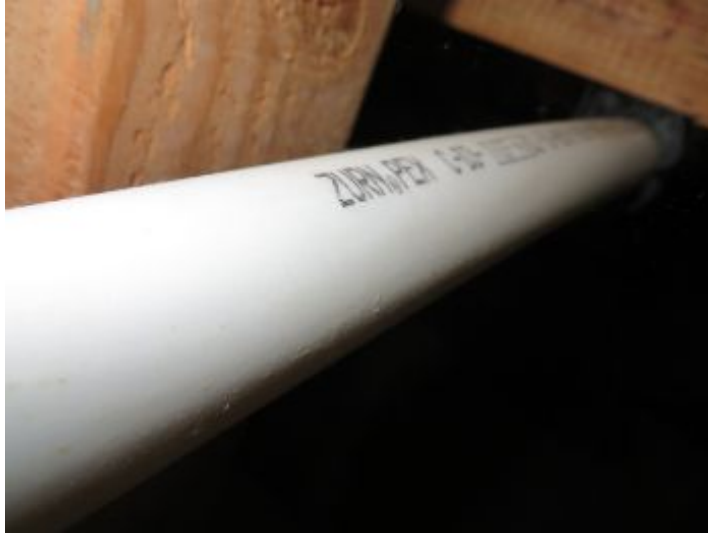
Zurn Pex plumbing. No sign of leakage or concerns at time of inspection.
