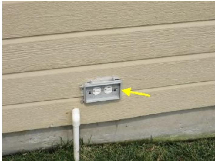
Exterior Outlet cover behind garage damaged.
