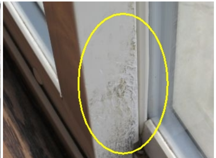
Sliding Door is scratched at the interior lower edge. Cosmetic only. Function is normal
