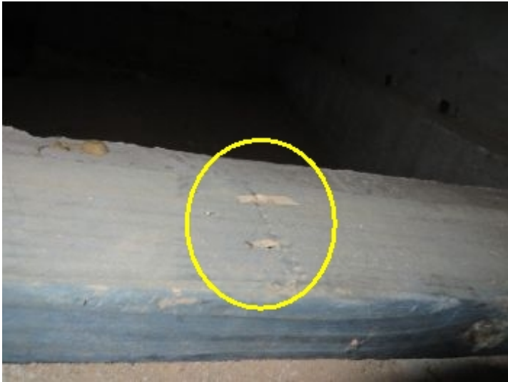
Nail marks where the support was removed from
