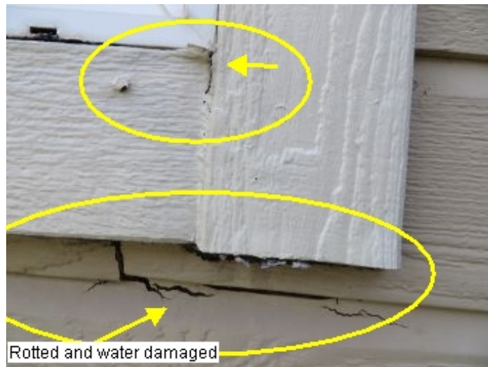
Siding under kitchen window is damaged at the corner. See photos. Recommend repair. Consult with licensed contractor on estimates/repairs
