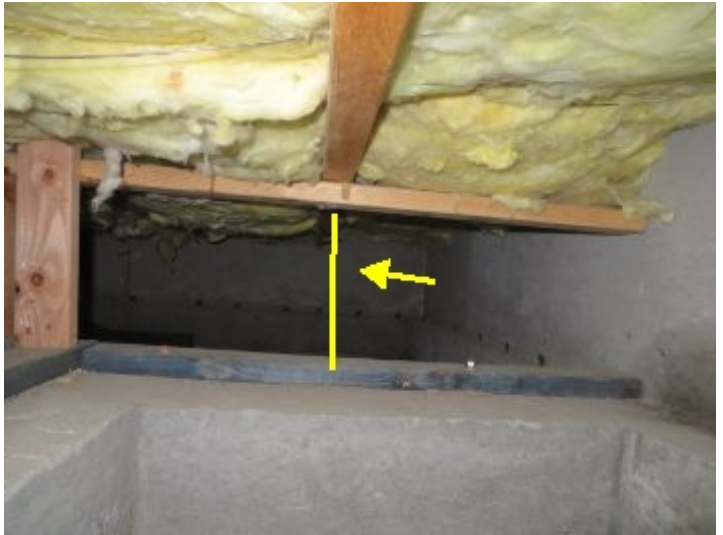
Support wall top plate board is missing support post. See photo. This is about 6 feet from hatch toward the front of the home. Someone has removed the vertical support board which helps support the long span of the floor joist. Sagging is beginning to occur. Need to add the vertical support again.
