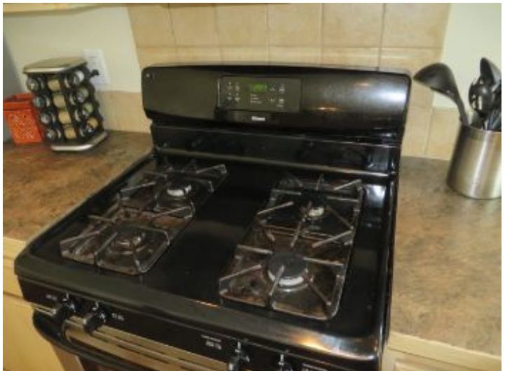
Safety Hazard- Stove Missing anti-tip brackets. This is needed to prevent injury or death. Recommend install prior to moving in.
