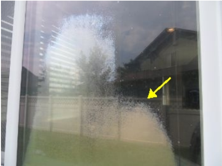
Kitchen window over sink (east side) has broken seal and fogging. Consult with window contractor on repair
