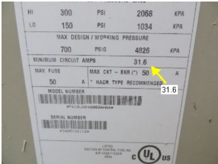
Minimum breaker according to label
