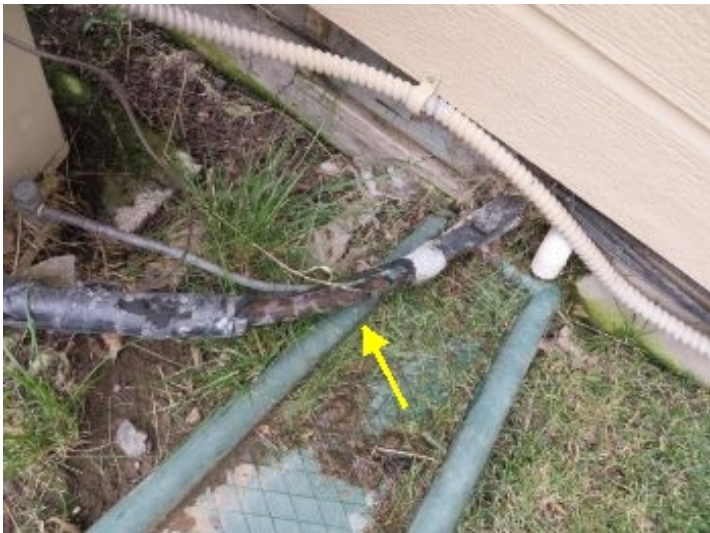
AC Unit refrigeration line insulation is damaged. This can cause damaged to the lines and unit and should be repaired.
