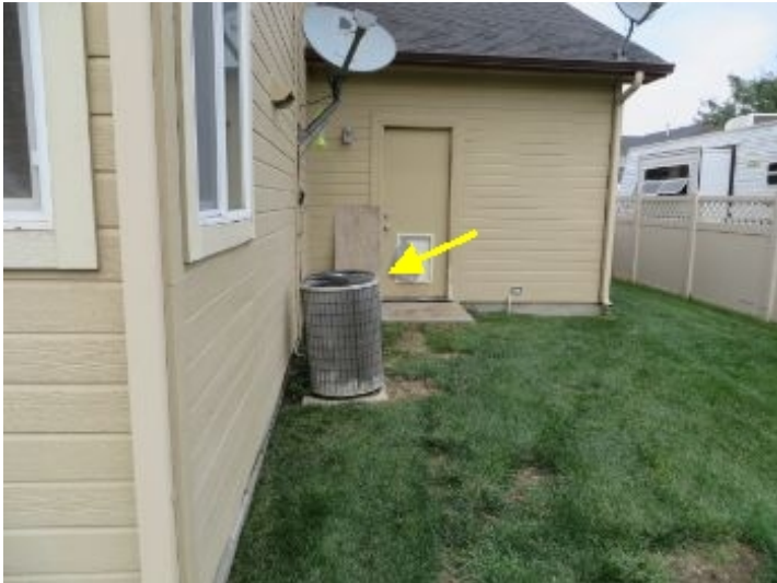
AC unit out of level. This can reduce the life expectancy of the unit and components. Recommend having leveled by licensed HVAC contractor
