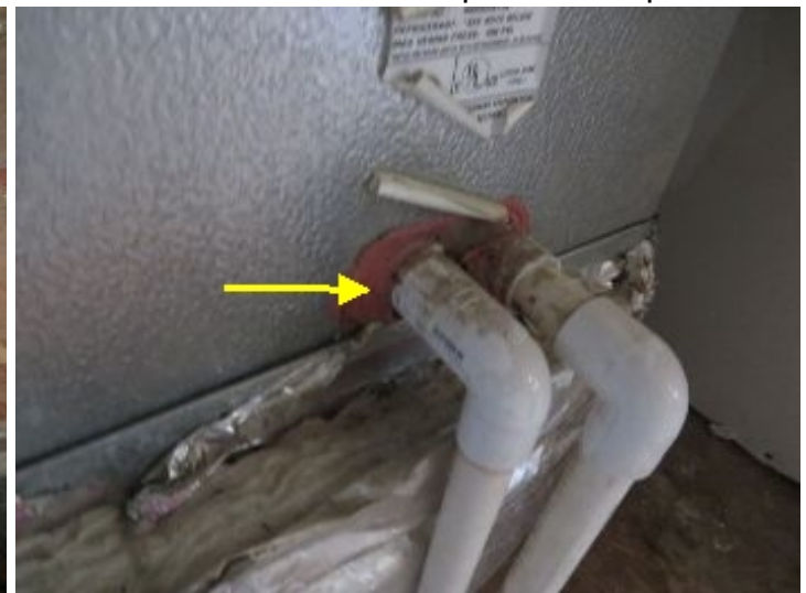
Condensate line has no water coming out
