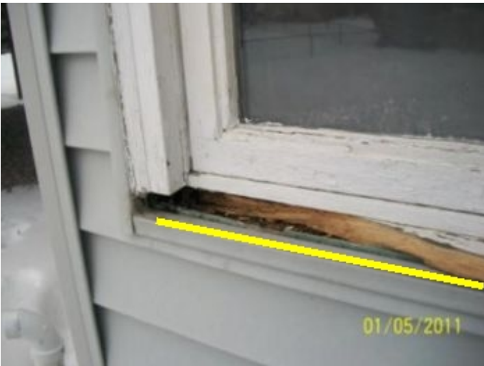
Extensive rot around window frames and sills
