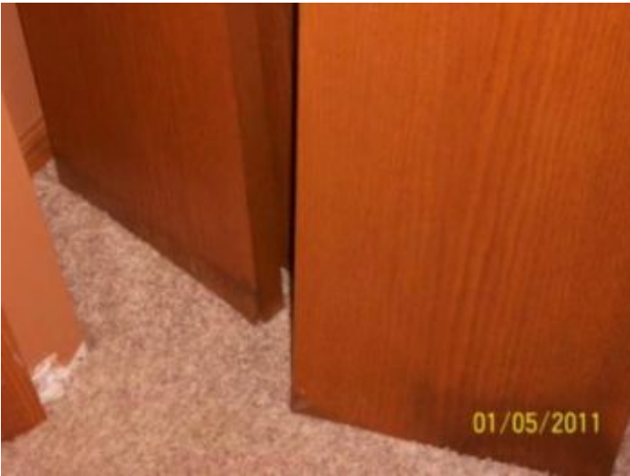
Bedroom Closet doors damaged
