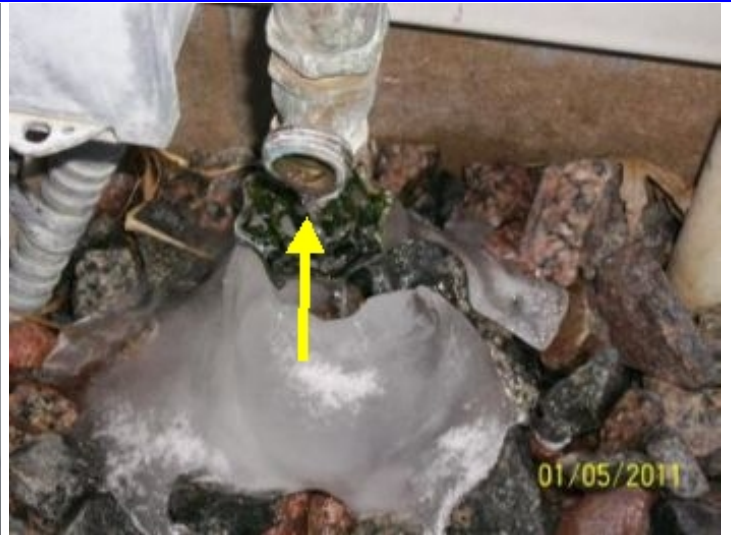
Hose Bib Leaking
