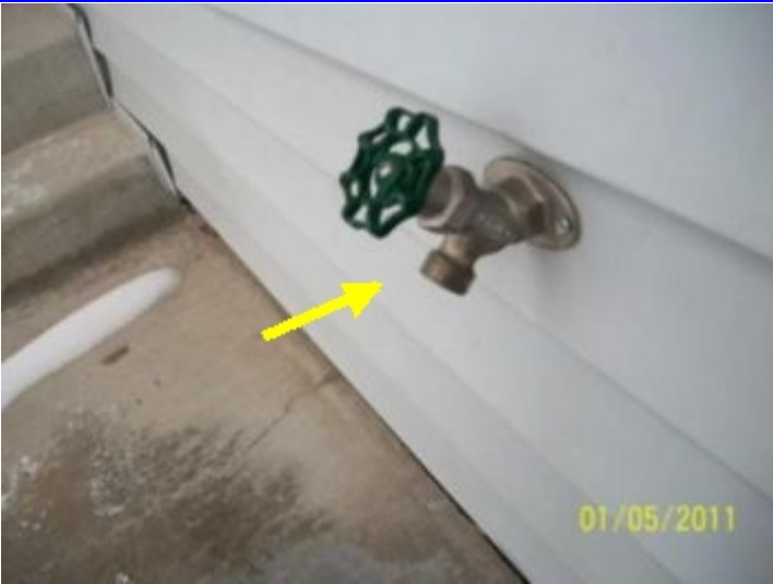
Need Anti-Siphon on exterior bibs
