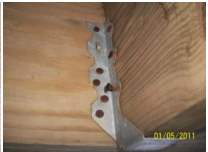
Joist hanger nails pulling out, rusting and not correct type
