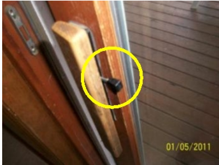
Door hardware/ lock damaged.
