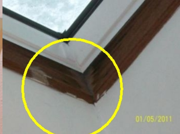
Skylight Moisture Staining. Area dry at time of inspection. Monitor
