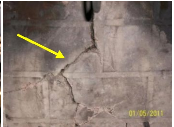
Rear wall of fireplace box damaged, needs repair for safety.
