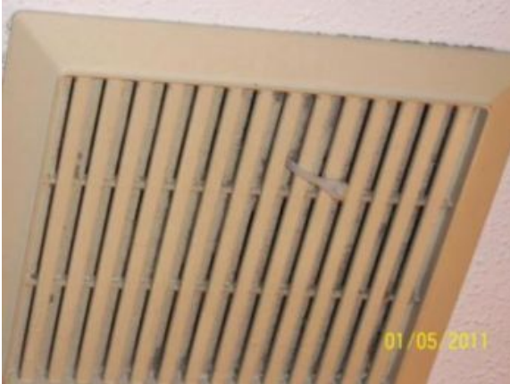
Clean bathroom fans
