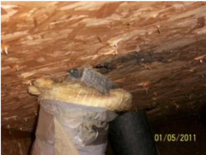
Exhaust fan not vented properly in attic. Moisture staining and sheathing deterioration noted.
