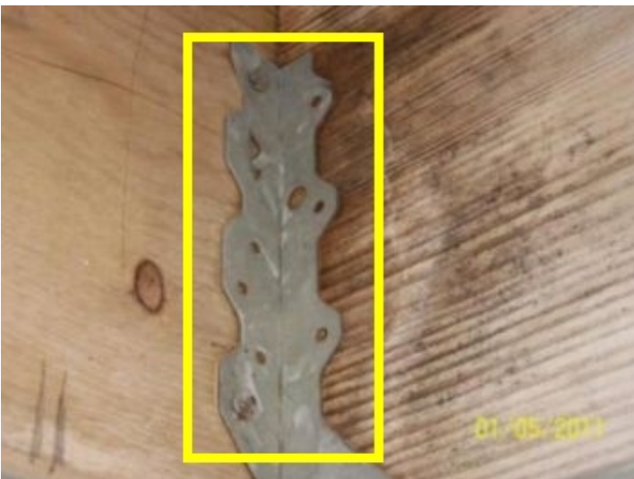
Safety Hazard- Deck Joist hangers missing nails. Recommend add needed hardware. Advise with contractor.
