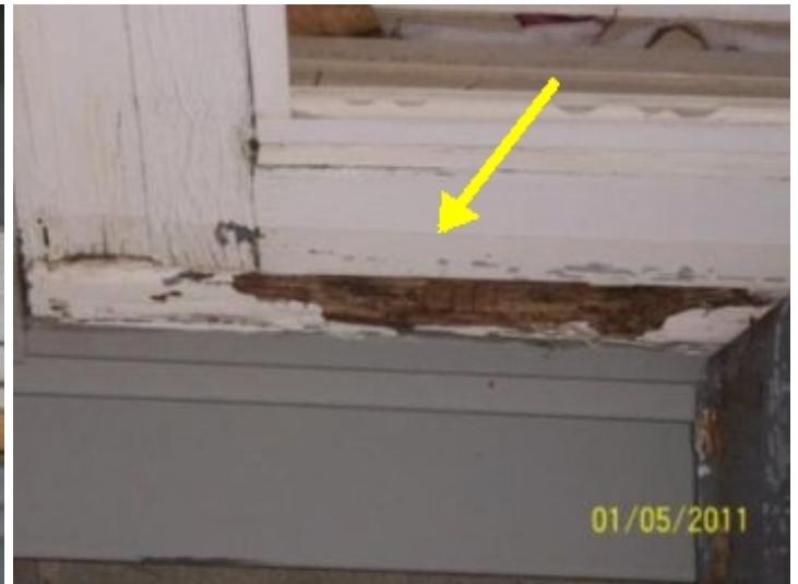
Extensive rot around window frames and sills
