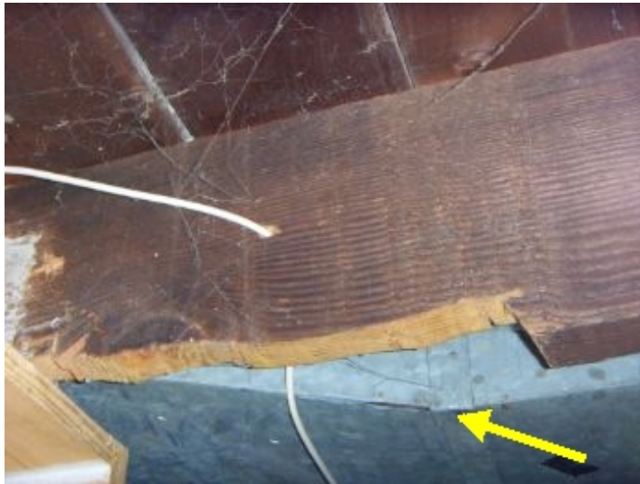
Joists Notched/Cut. This can pose a structural issue or cause future damage if left unsupported. Recommend consult with contractor on adding additional support or repair.
