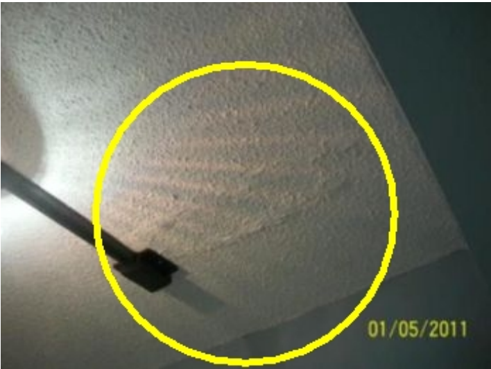
Prior Moisture Ceiling Staining- Tested Dry at time of inspection. Monitor for leaks!
