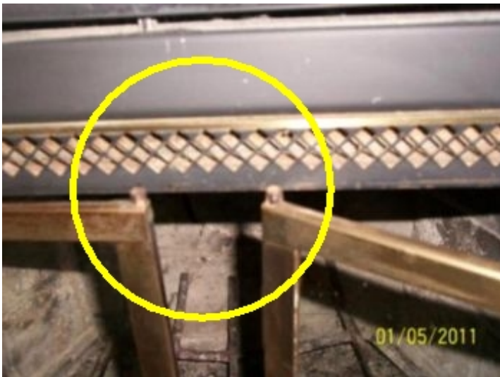
Fireplace Glass/Doors need cleaning & improvement
