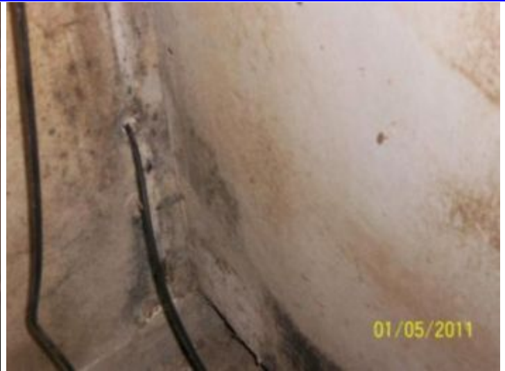
Possible organic substance noted. The United States Environmental Protection Association (EPA) states, "If you believe that you may have a hidden mold problem, consider hiring a professional." (Brief Guide to Mold, p.14, EPA). If any area of the residence is suspected of having organic growth, or any member of your family or household is sensitive to mold, we are lab-certified to conduct a Mold Inspection / Sampling to identify the types of mold (or any other airborne allergens) present. If necessary, we are also lab-certified to perform radon, meth, asbestos and other environmental testing services. See: www.IdahoHomeInspectors.biz/rates for more information.
