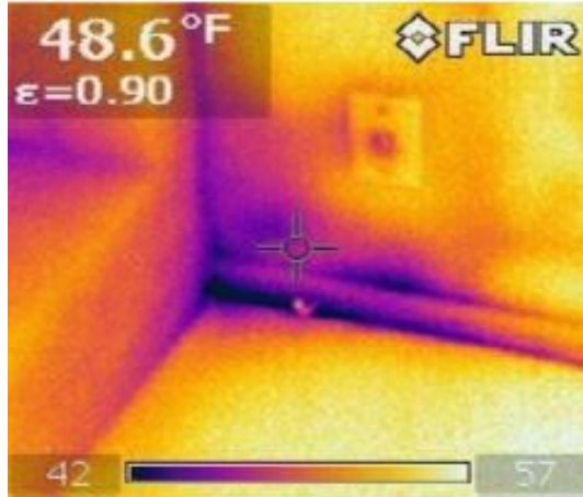
Low level of missing insulation in bedroom upper level
