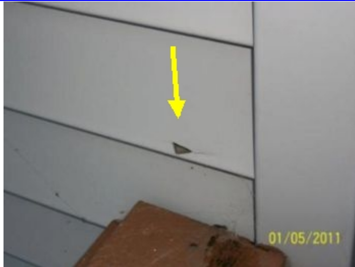
Vinyl siding damage. Recommend repair or replacement of damaged sections to keep moisture and insects from harming structure.
