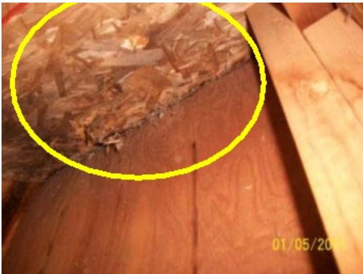
Evidence of past or present leaks, dry at time of the inspection. Monitor for leaks &/or have roofing contractor evaluate.
