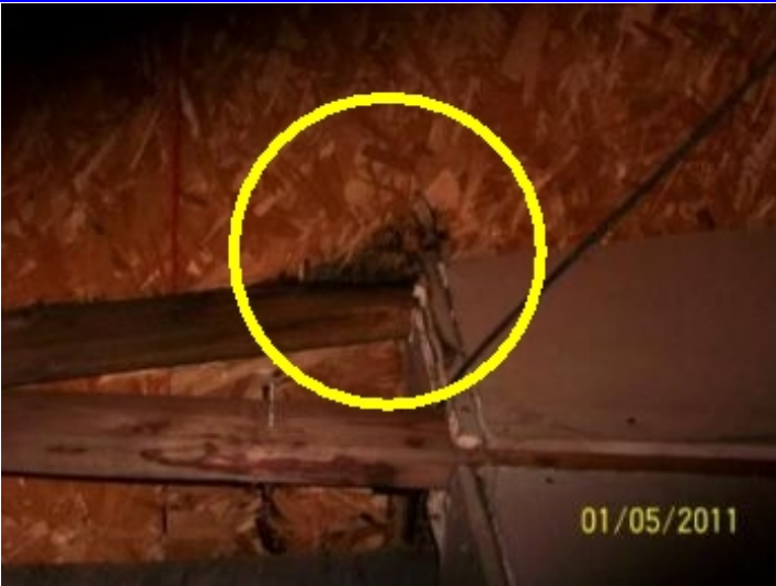
Evidence of past or present leaks in garage ceiling/wall, dry at time of inspection. Monitor this area, or have it evaluated further.
